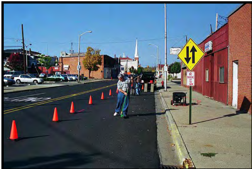
Figure 5 Courtland Street (Site 3)
